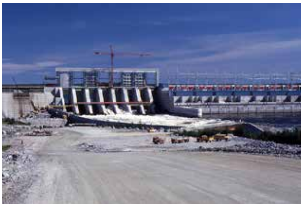
(1993) Hydro-Quebec's La Grande project dam flooded thousands of hectares on Cree land, displacing all Cree in that area. Photo: Langelle/GJEP-GFC & PhotoLangelle.org
